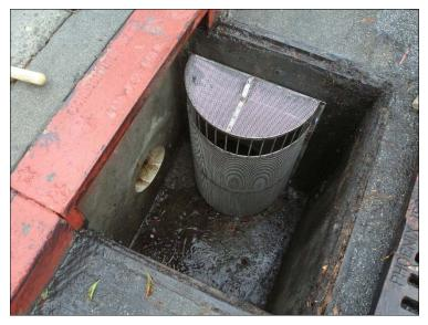
Figure 2.2. Example small full-capture device used as a monitoring site.
